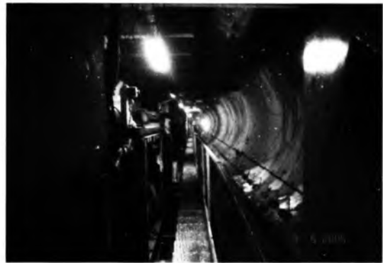
Photo -2 : Segmental lining at ILPS
